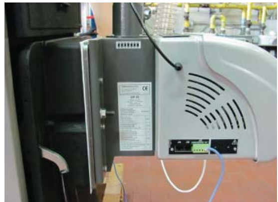
Fig. 26 Fixing of the burner
