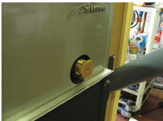
Fig. 27 Brass reducer
